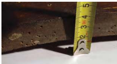
▼ Fig. 4. Lacuna in the crossbar produced as a result of the weakening of the wood due to xylophagous insects.
