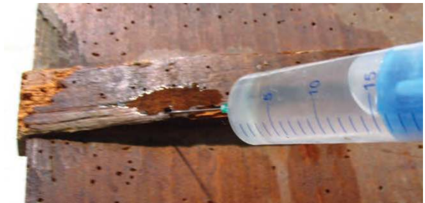
▼ Fig. 7. Applying the insecticide on the back of the panel.
